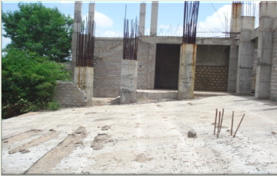
Dismantled RCC slabs and stage beam of Auditorium at JNTU, Anantapur (10 August 2012)
